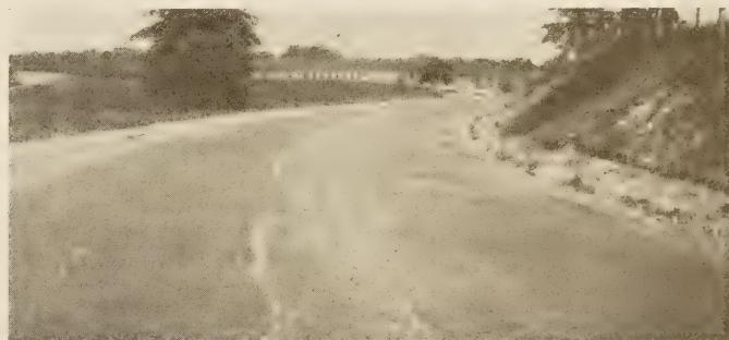
FIG. 8.—Test 18 shows the distribution of traffic on 22-foot bituminous macadam road at an 11° 30' curve which has a crowned super-elevated section. Vehicles traveling on the outside of the curve crowd toward the inside to take advantage of the favorable slope and reduce curvature, and in the absence of a center line there is nothing to counteract this tendency
